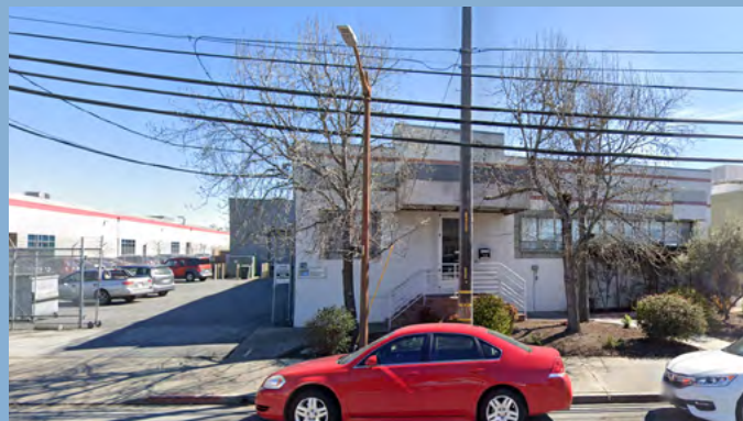
ISC's former headquarters at 950 Charter Street in Redwood City, California. We didn't even get to say a proper goodbye.
